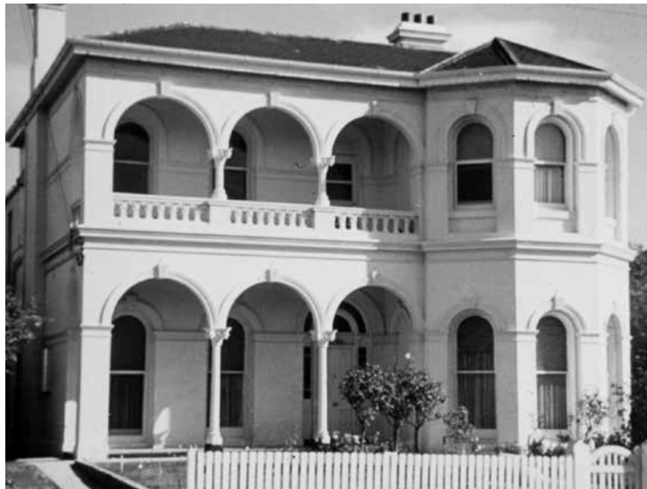
49 Mathoura Road, Toorak, Melbourne. Headquarters of the Society 1950-55. The lower bay window, right, was that of the lecture room and the windows to the left of the front door were those of the library. The upper storey was the residence of Dr Geoffrey Kaye
