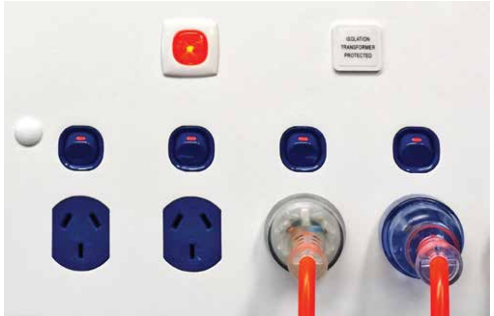
Diagram 5: Operating Room line isolation monitor (LIM) protected outlets from an uninterruptible power (blue outlet)
