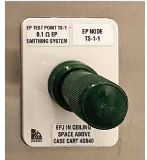
Diagram 3: Cardiac protected electrical area earthing test point
