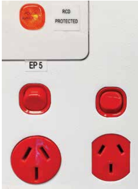
Diagram 4: Operating Room RCD outlets from a generator power supply (red colour outlet)
