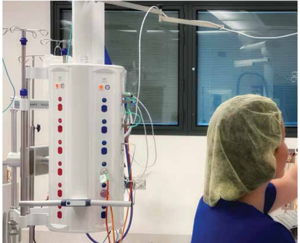
Operating theatre pendant with both generator and UPS electrical outlets
