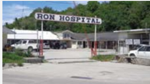
The Republic of Nauru Hospital entrance
